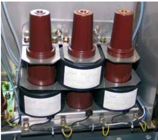
Bottom view of toroidal type current transformers on external-cone cable plug-in terminals (T2 function)
