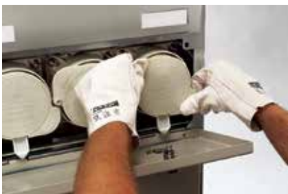
Do not turn the gripping surfaces but use them to pull the fuse out
